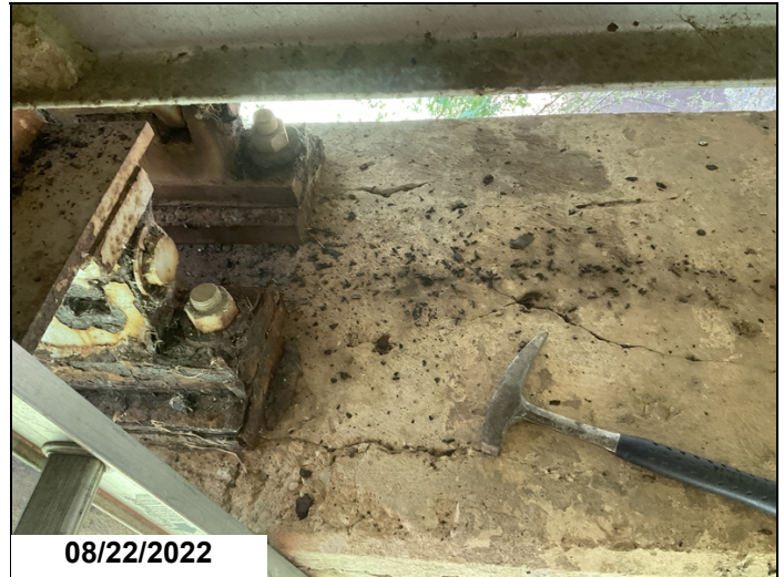
Bent 4 Rt cracking and delaminating concrete in the top of the cap.
