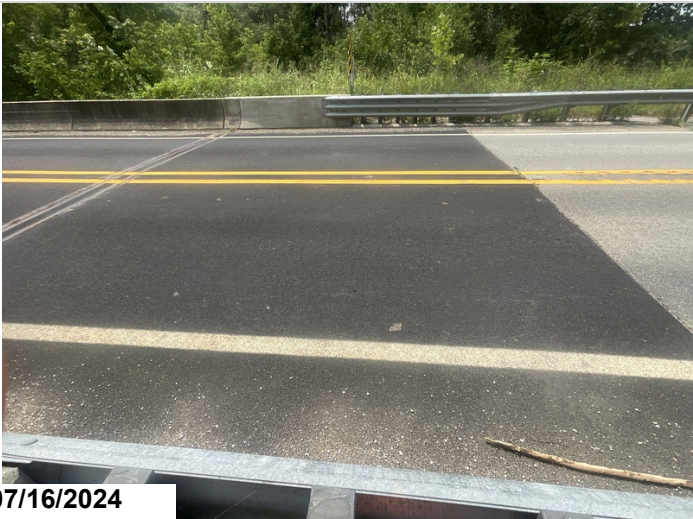
West approach slab. New polymer wearing surface.
