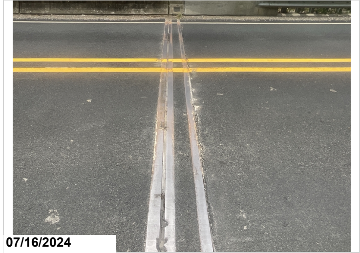
Top of Abutment 1 backwall. Polymer wearing surface.
