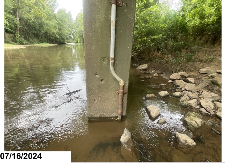
Bent 2, Column 1 has minor shallow spalls adjacent to the water quality testing brackets.
