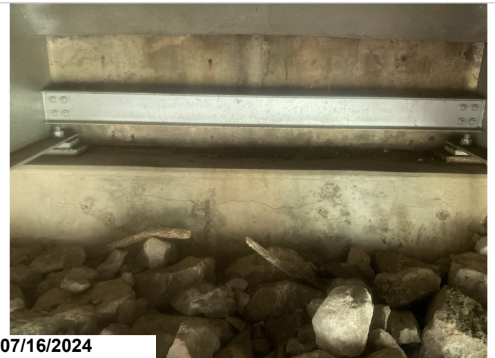
Abutment 2 cap, Horizontal crack approximately 1/16" wide.
