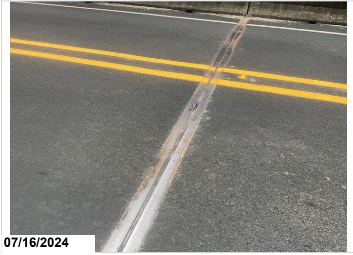
Expansion joint seal over Bent 4. Typical.
