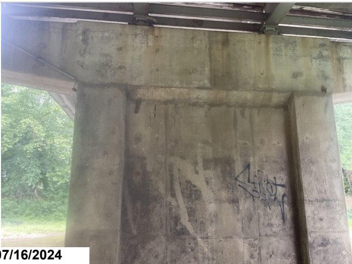
Bent 2 back face has a 12" spall and a 2' delaminated area in the web wall.
