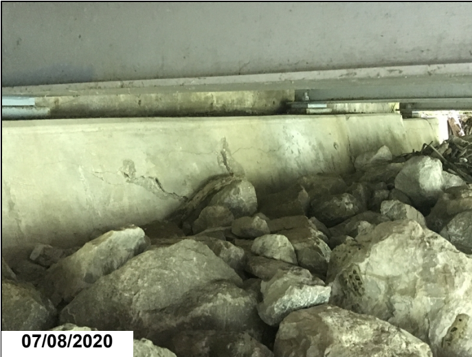
Abutment 2 cap has delaminated areas and spalls with exposed reinforcing steel.
