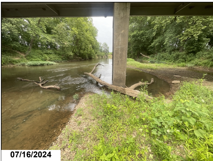
Bent 3. Drift accumulation.
