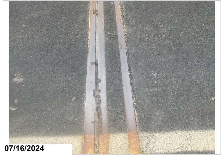
Abutment 1 expansion joint seal.
