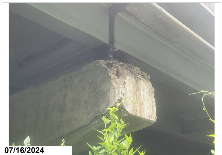
Bent 5. Right end of cap. Soft deteriorated concrete with exposed reinforcing steel.
