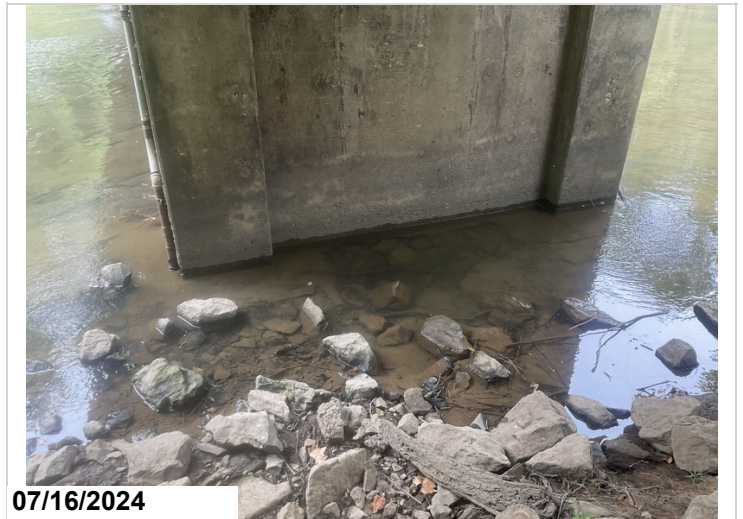
Top of Bent 2 footing exposed.
