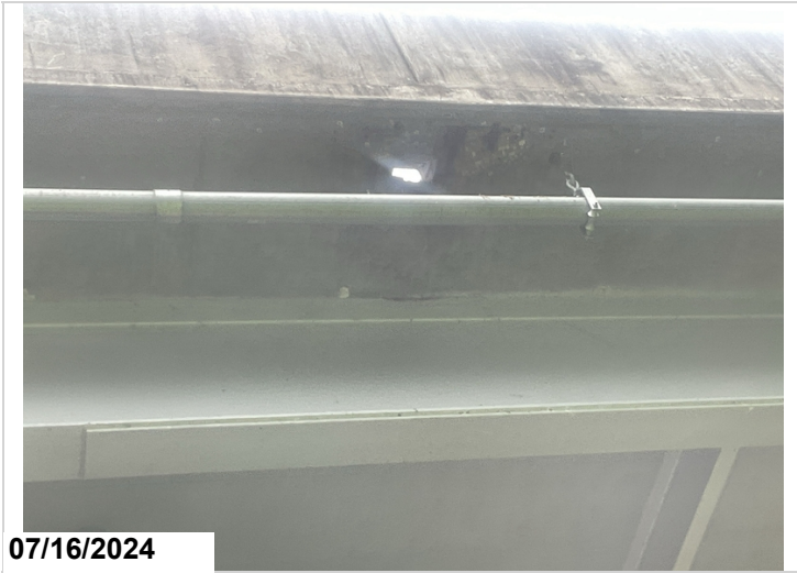
Span 3, Right side, Deck undersurface has Spalls with exposed reinforcing steel adjacent to the deck drains.
