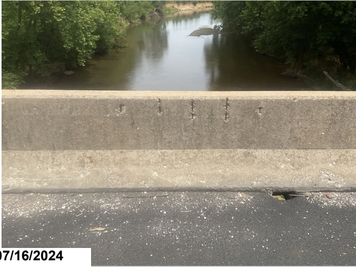
Left Parapet. Spalls with exposed reinforcing steel.
