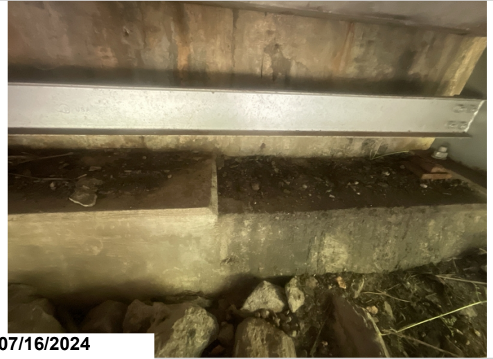
Abutment 1. Debris on cap.
