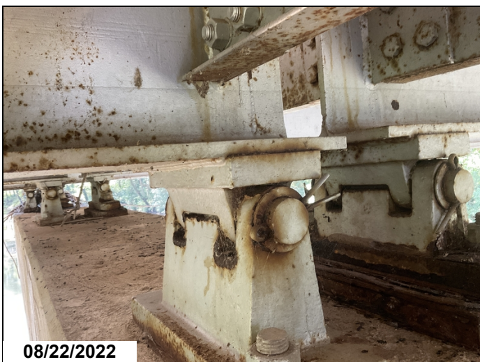
Bent 3 bottom flange misalignment from active corrosion between the masonry plate and the expansion bearings.
