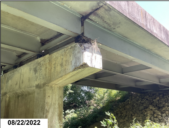
Bent 5 Rt concrete deterioration with exposed reinforcing steel.
