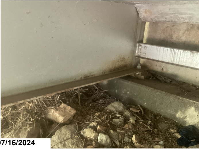
Abutment 1, Girder 4 has areas of corrosion showing through the paint system.
