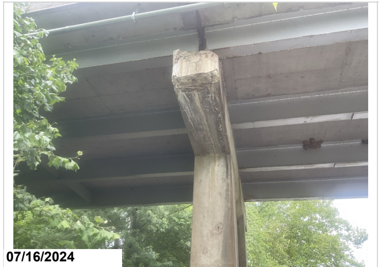
Right end of Bent 2 cap. Concrete deterioration with exposed reinforcing steel.
