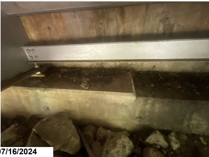
Abutment 1. Debris on cap.
