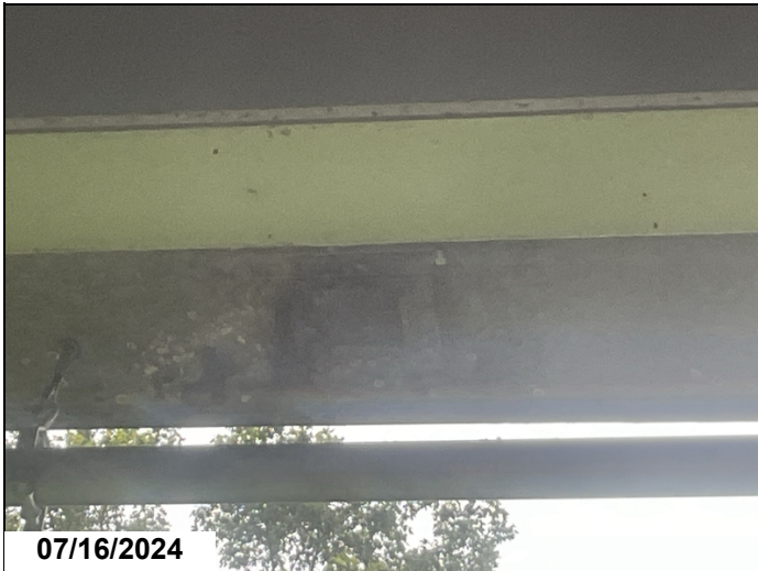
Spalls with exposed reinforcing steel next to the drains. Span 3 Right.
