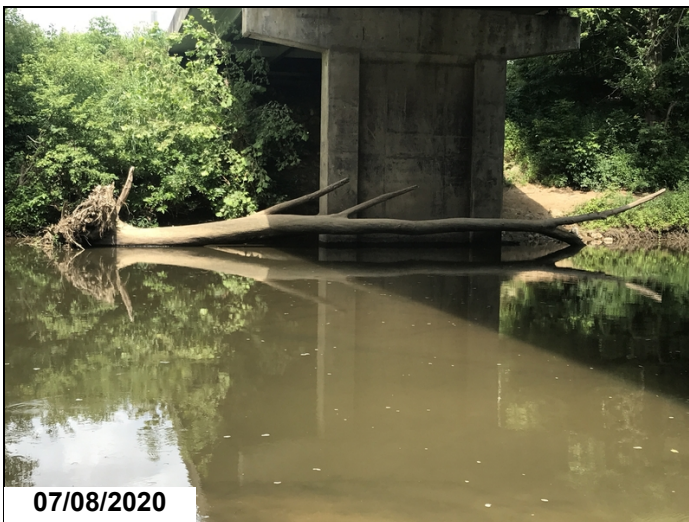
The channel has a tree wedged against bent 2.
