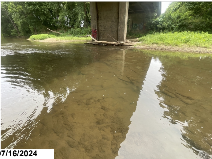
Solid rock Channel exposed under Span 2.
