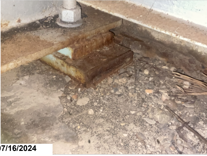
Abutment 1 Girder 2, fixed bearings have active corrosion with flaking rust.
