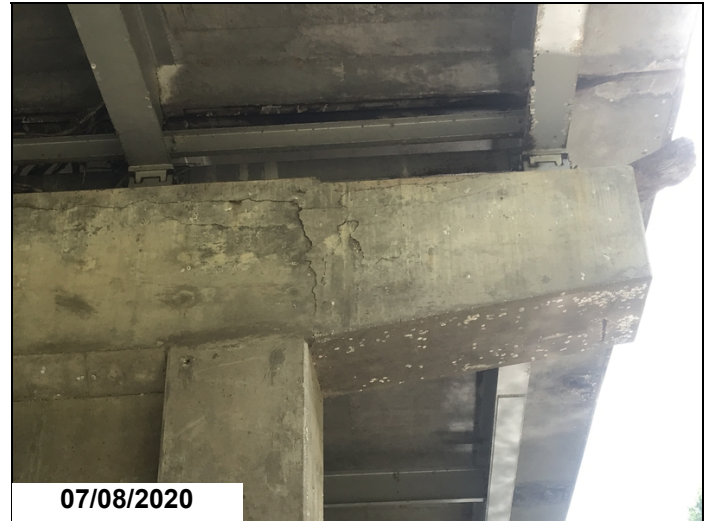
The intermediate bent caps have moderate width horizontal cracking, concrete deterioration with map cracking, and spalling with exposed reinforcing steel.
