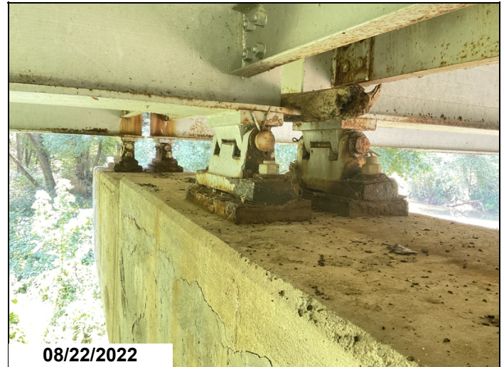
Bent 4 bearings with active corrosion and pack rust.
