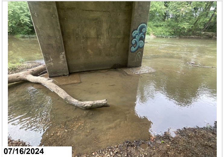
Bent 3 footing exposed.
