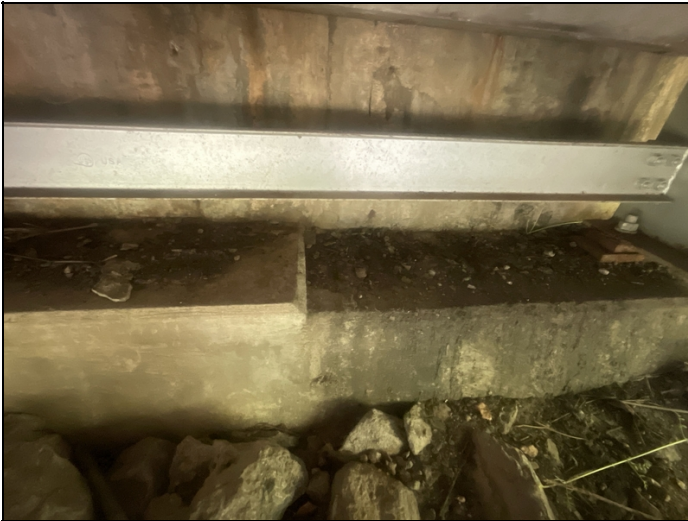
Abutment 1. Debris on cap.
