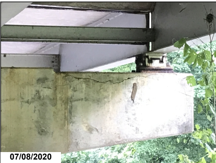
Bent 2 cap-Wide horizontal cracking.
