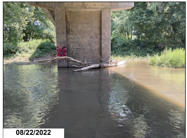
Bent 3 drift accumulation.
