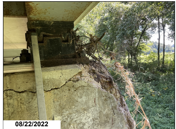
Bent 5 Rt top of the cap delaminating with loss of bearing area and exposed reinforcing steel.
