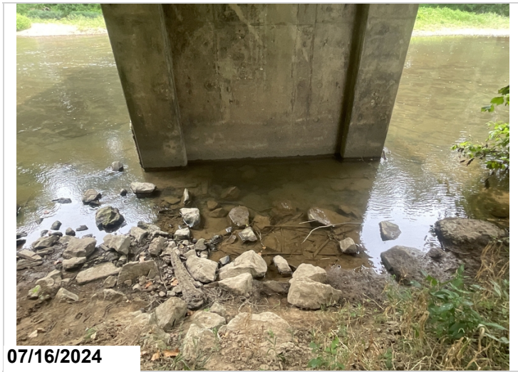
Bent 2 footings exposed.
